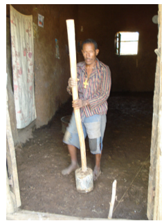
Compacting dirt floor
